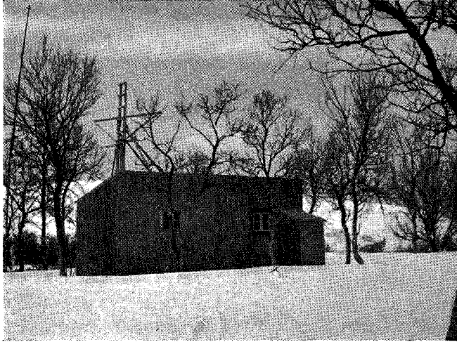
Fig. 20. Transmitter hut with antenna arrangement.
